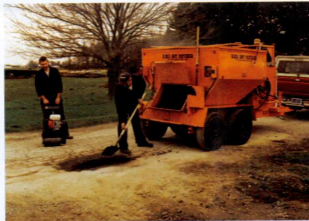
Available in truck or trailer-mounted models, hotboxes (and recyclers) help cut back on waste and the costs associated with it. Before hotboxes contractors had a brief time to use the hot mix before it began to harden on them. Heated hoppers give contractors more hours in a day to work.
