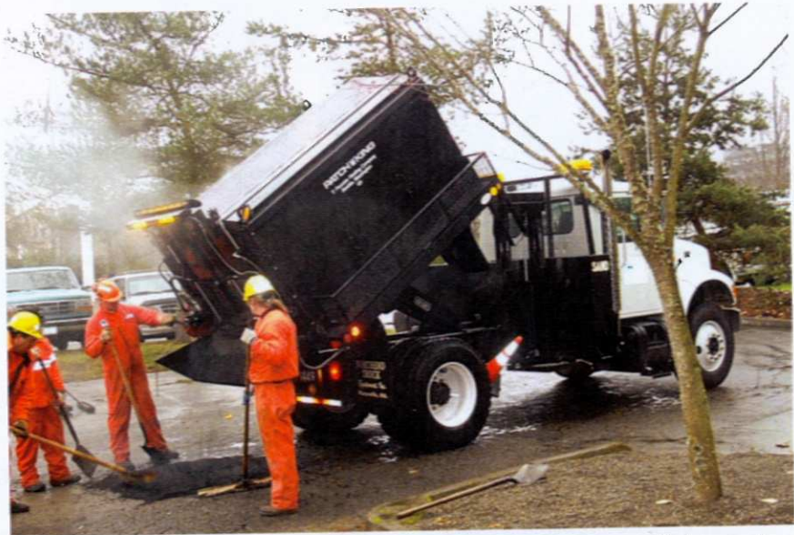
Hotboxes allow contractors to keep mix heated all day or overnight, which saves on costs and reduces waste.
