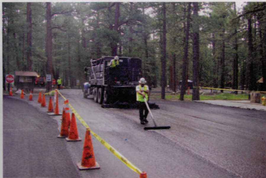
Most National Parks consider micro surfacing (shown here), slurry surfacing, chip sealing and other pavement preservation processes to be very environmentally friendly.
