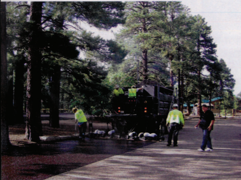
The flexibility of pavement preservation processes, such as micro surfacing, provides contractors the option to use alternative treatment combinations when job parameters change.
